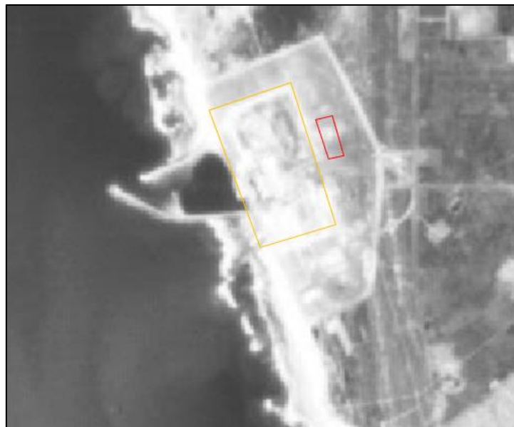
Figure 19: 1989 aerial photograph (Job 929, Strip 003, photo 02216) showing Koeberg Nuclear Power Station. The orange box shows the location of the main plant site, while the red box shows the location in which the car park lies. It is clear that the surface has not yet recovered to look like virgin veld.
